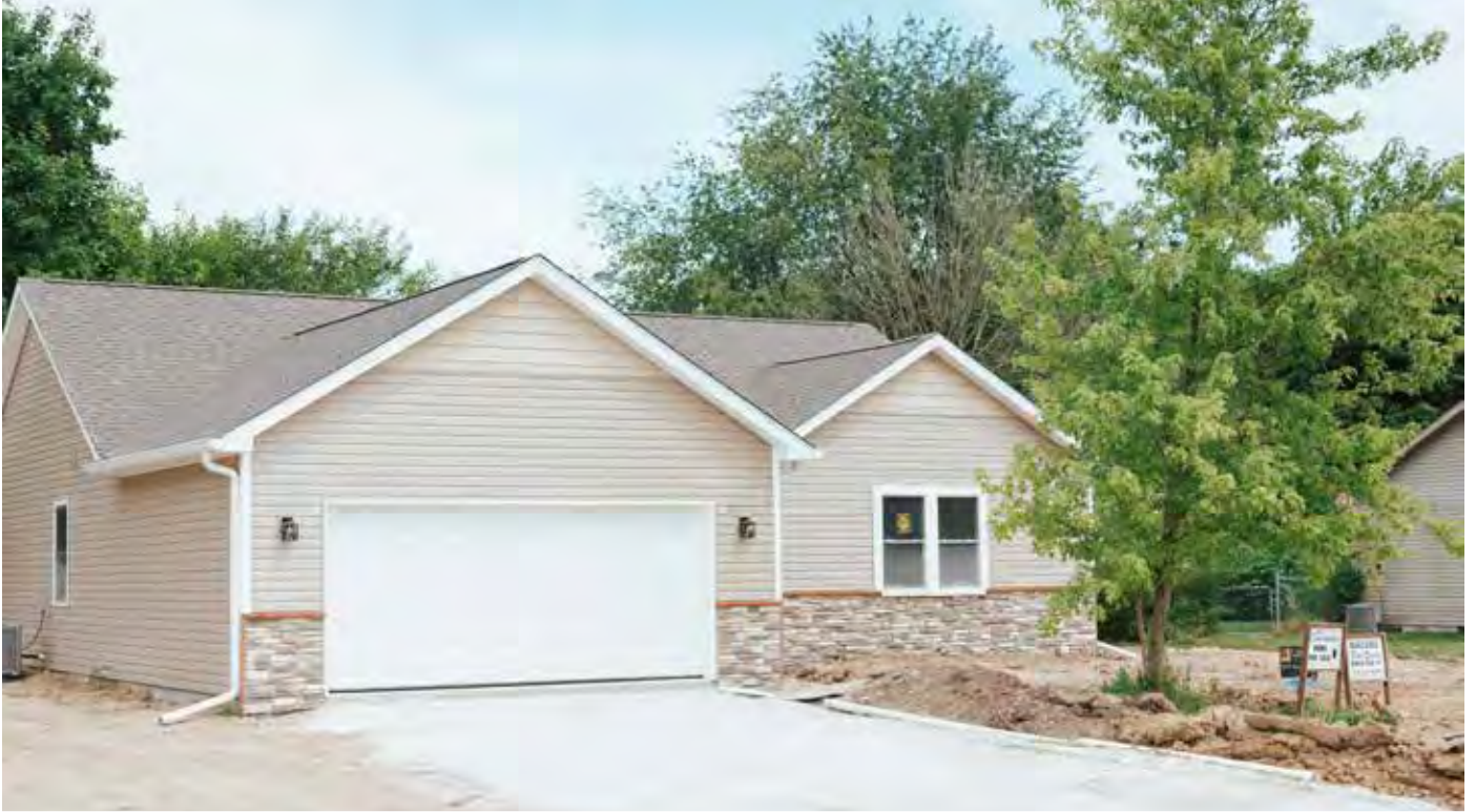
A home recently constructed in Heritage Lake.
