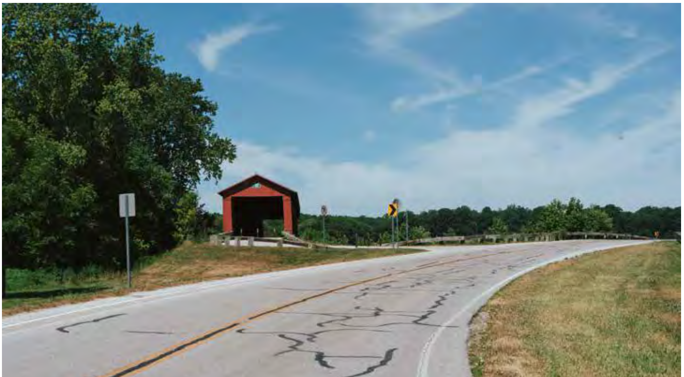
Houck covered bridge over Big Walnut Creek along W CR 550 S and N CR 500 W.
